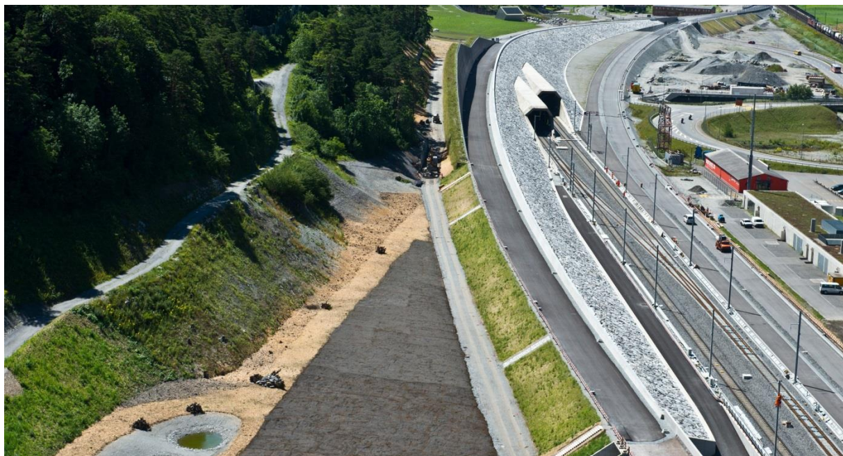
Figure 6.2 Completed Erstfeld Tunnel Staggered Portal with road over and headhouse
